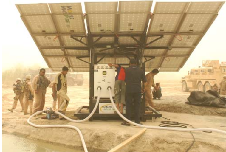
Marines and members of the Zobai Tribe set up solar powered water unit near Fallujah.
